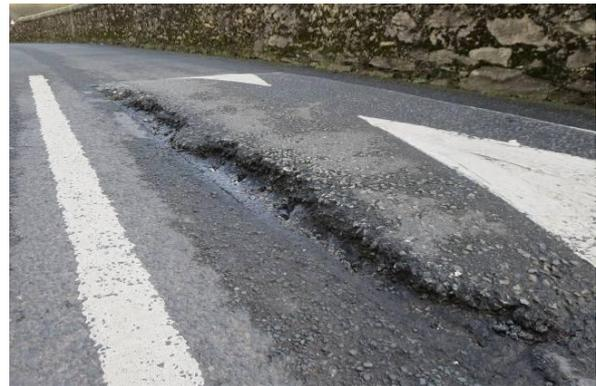
Two weeks before Christmas new humps were installed in Nefyn but the legal markings were only painted last week. For five weeks, black faintly marked humps were virtually invisible on dark wet nights. Anecdotal of reports said vehicles were bouncing into the air - what hidden damage was caused to tyres and steering of these cars? The new humps are already crumbling at the edges.
