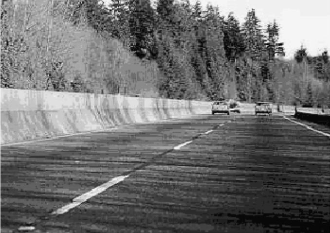
**Figure 10.** Paddles at angles less than 20 degrees appear to present a solid screen from the driver's view. (Courtesy glaregaard.com)
